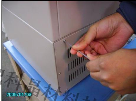
2. Find out the main circuit where the fuse locates and then, uninstall the fuse.
